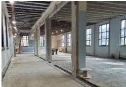
Max W & Maileen Brown Family Hall First Floor Renovation
