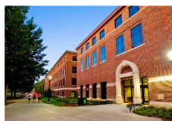
Mechanical Engineering Building Renovation
