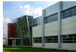
Birck Nanotechnology Center Clean Room Modernization, Related Renovations and Equipment Purchases
