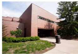
Whistler Hall of Agricultural Research Mechanical System Renovation
